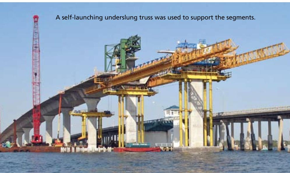
A self-launching underslung truss was used to support the segments.
