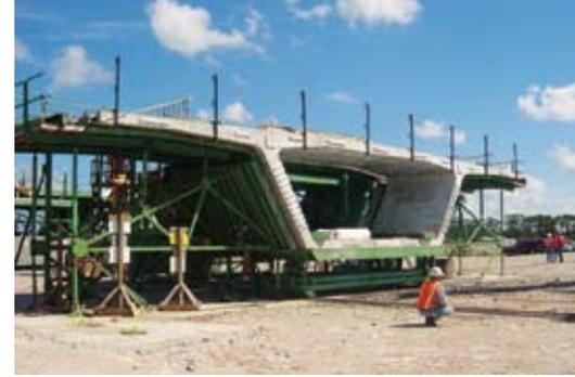
Typical segments were 10 ft long, 10 ft deep, and 61 ft wide, weighing about 80 tons.
