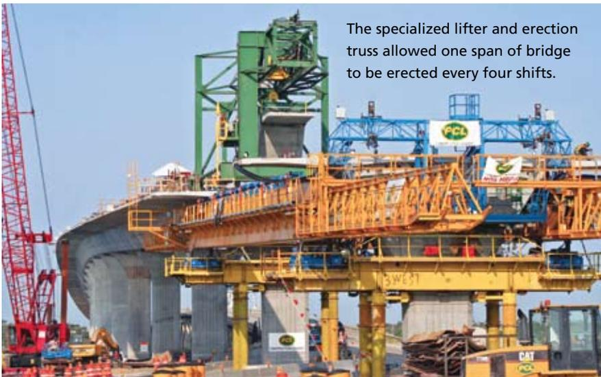
The specialized lifter and erection truss allowed one span of bridge to be erected every four shifts.
