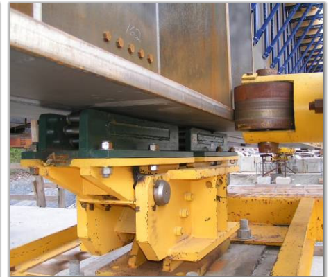
roller brackets and guide system at piers
