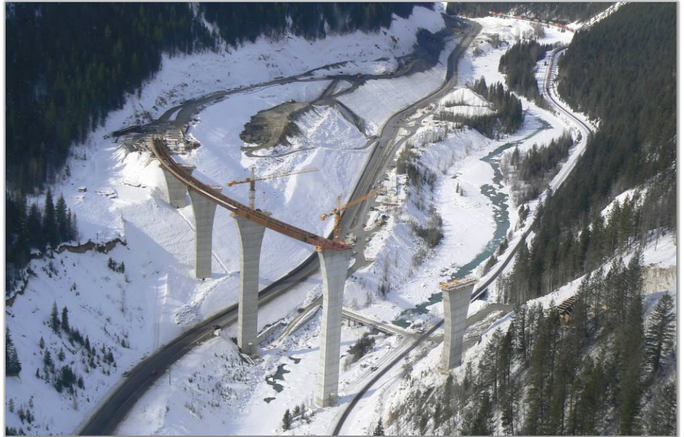
the first set of girders reaches the fourth and tallest pier in February 2007
