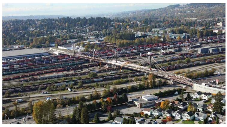
ushing a nearly 5,000 metric ton steel superstructure across a span of 580 metres and over railway tracks is no easy feat. But that is exactly what had to be done for Port Coquitlam's new Coast Meridian Overpass.
