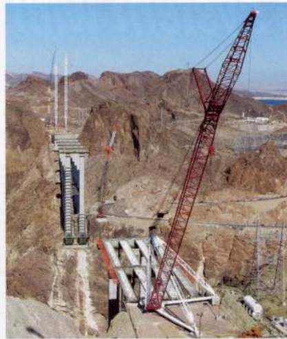
Left: The interim delivery system in the foreground, with the new high-line shown behind
