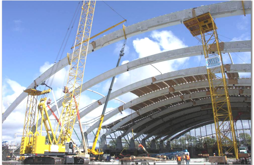
erection of the self-supporting composite arches on temporary shoring towers
