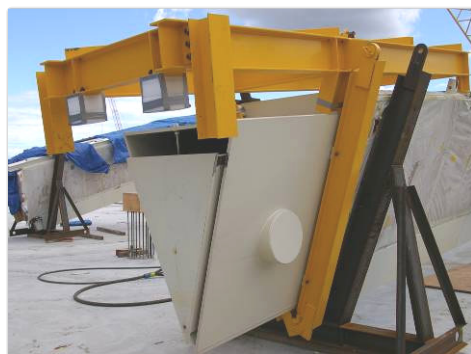
jacking support frames take full weight of arch until the arch is complete and end plates are grouted
