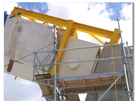
jacking support frames take full weight of arch until the arch is complete and end plates are grouted
