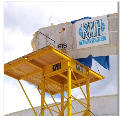
erection of the self-supporting composite arches on temporary shoring towers
