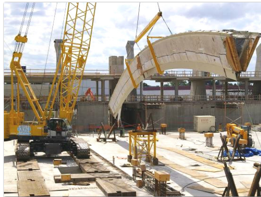
lift of 40 ton section employed specialized lifting devices
